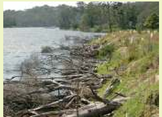
Wattles have been keyed into the eroding bank and planted out with shrubs and trees.
